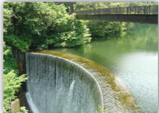
Gambar 4. Tipe Lengkung Sabo Dam sumber : Technical standards and guidelines for planning and design of sbao structures, JICA,Juni 2010
