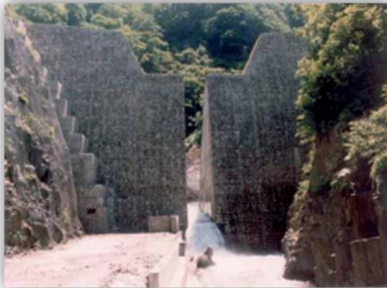
Gambar 6. Tipe Permeable Sabo Dam
