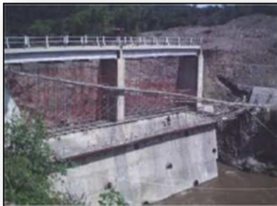
Gambar 7. Tipe Permeable Sabo Dam
